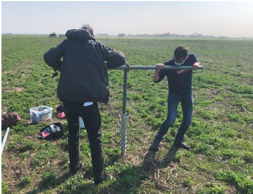
Figure 12: installation of the screw foundation
